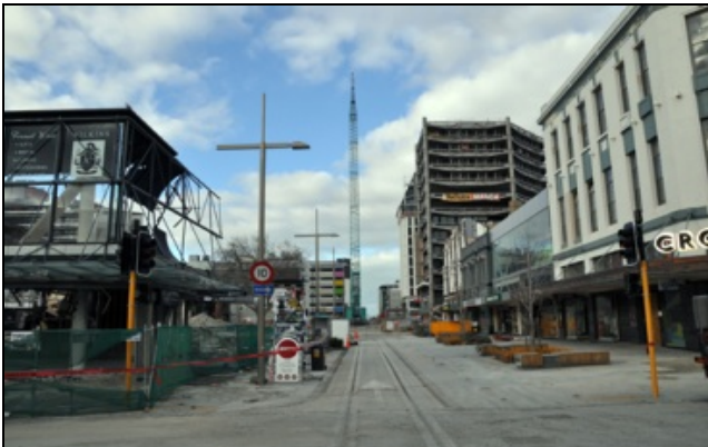
Rebuilding Christchurch's Central Business District.
